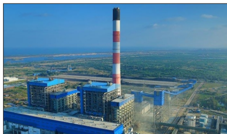
Power & Energy Sector
